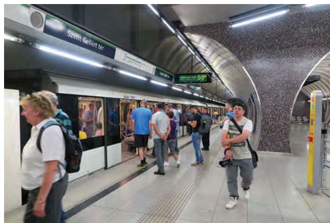
The ultra-modern Szent Gellért tér station and train on line M4 of the Metro. Each station has a different decoration - in this case impressive mosaic tiling.
